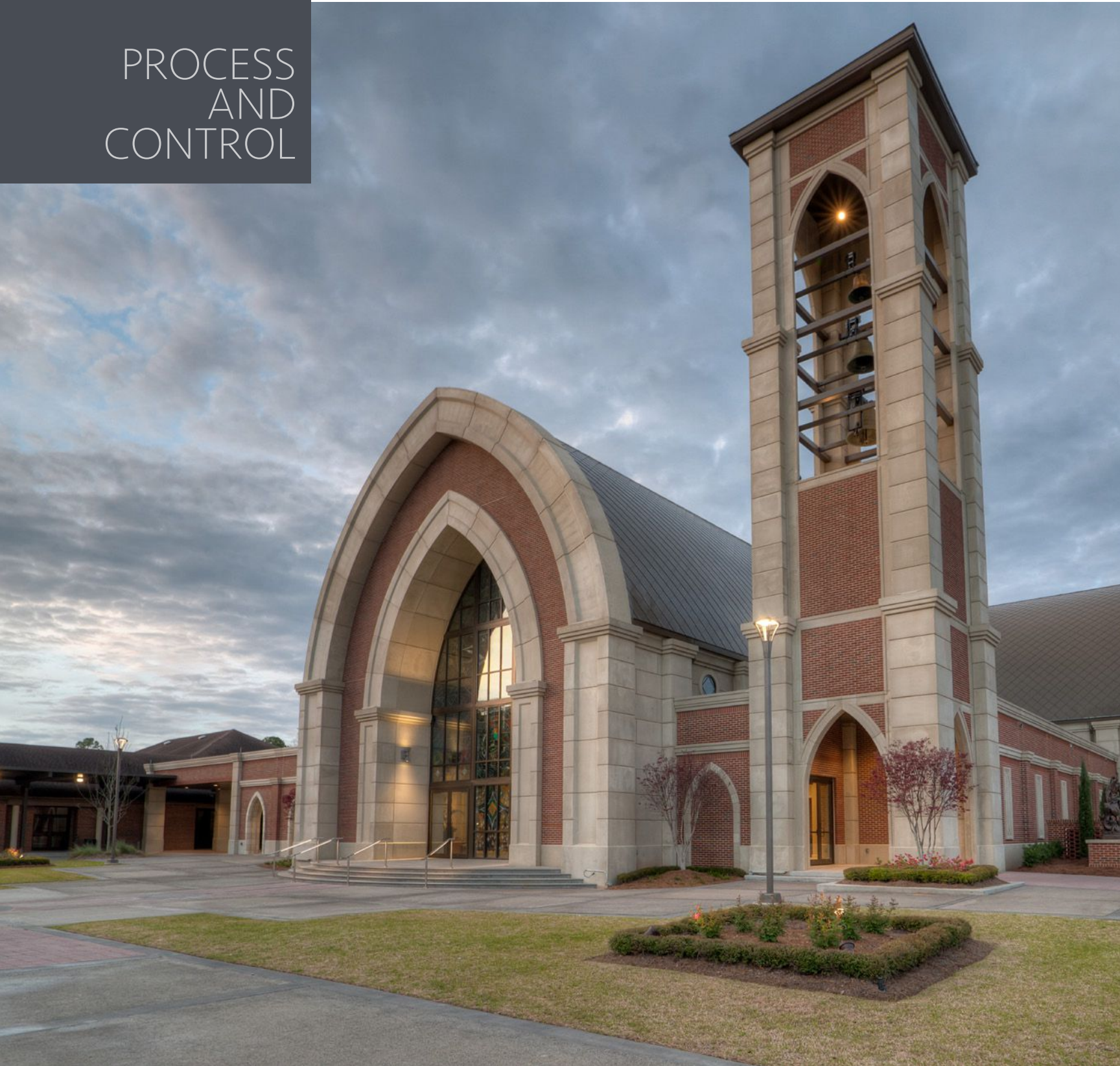
Mark Ledkins, vice president, operations, Southern Division, GATE Precast, reviews mock-ups with visitors. The result was the beautiful St. George Catholic Church in Baton Rouge, La. Photos: GATE Precast and toddlandryphotography.com.
