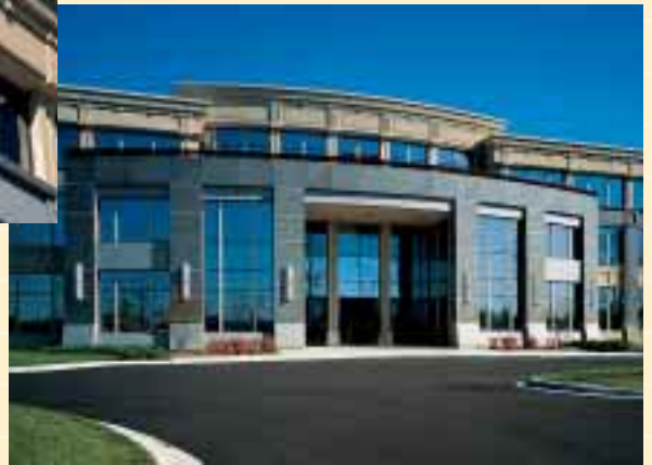
Holley Court Parking Facility in Oak Park, Ill., features precast concrete details that add both character and interest to the cornice and façade. The goal was to suggest residential rowhouses rather than a parking structure. Photo: © Steinkamp/Ballog Chicago
