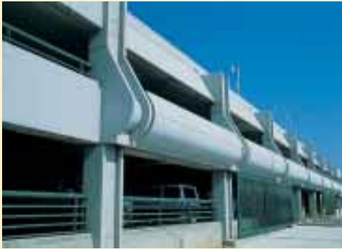
Large bullnose components added to the parking structure at the Hyperion Wastewater Treatment Facility provided a distinctive visual element that tied it to the other buildings in the project without mimicking their exact look.
